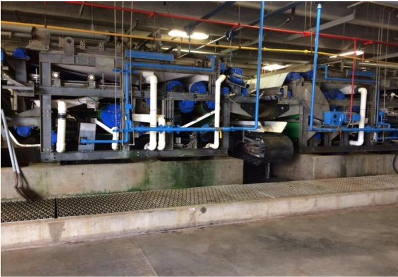
Wasted biosolids from the activated sludge process are retained in the sludge holding tanks for further compaction. The thickened sludge, 1% solids, is then applied to the belt presses for dewatering prior to final disposal. The belt presses remove an average of 8-9 dry tons of solids per day from the waste biosolids.
