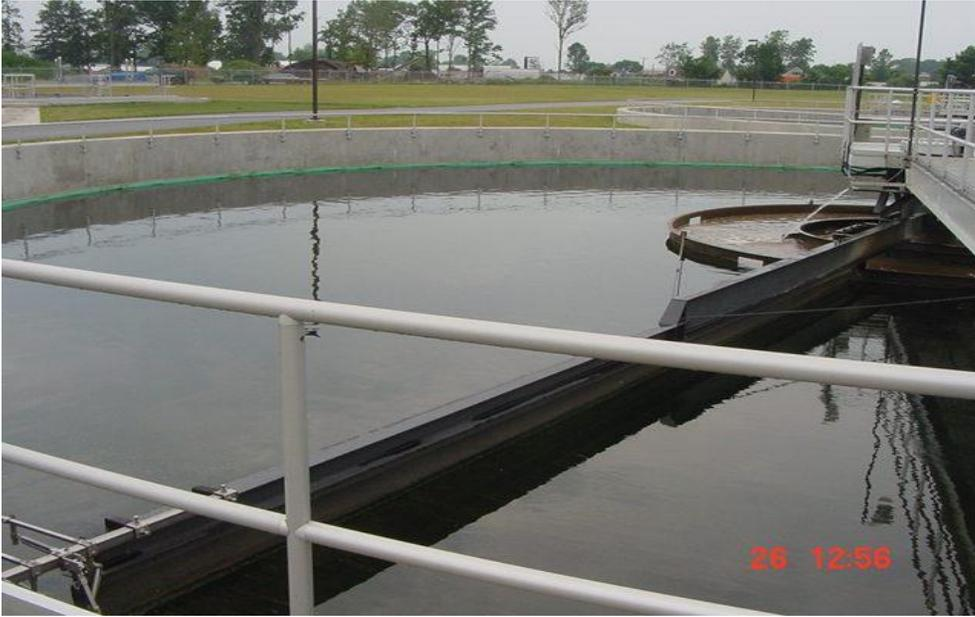
In the clarifiers, biological growth is settled from the wastewater and a portion is returned to the oxidation ditches to maintain the process. After clarification, the wastewater is piped into the disinfection chamber.
